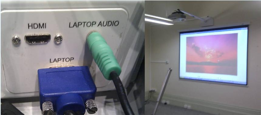
Due to distance limitations of HDMI signal, high quality cables are needed to be installed for long cable lengths. Where installation points are over 15mtr, a HDMI over Cat5/6e system is needed. There are also products that can covert HDMI signals back to Analog VGA signal. So if your new laptop doesn't connect into your existing system, you are able to complete a minor upgrade without the need to replace projectors and cabling. Contact us to find the best solution for your needs.
